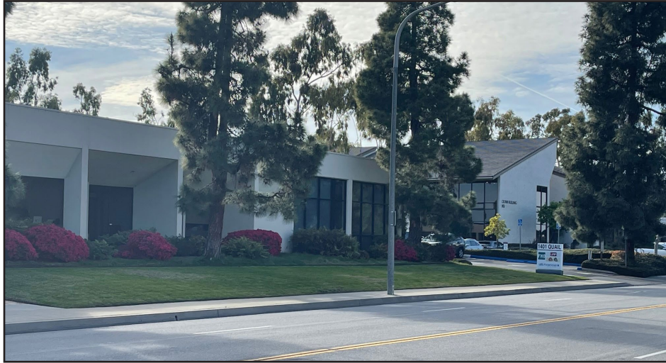
Photo 1. From Quail Street looking southwest across the project site.
